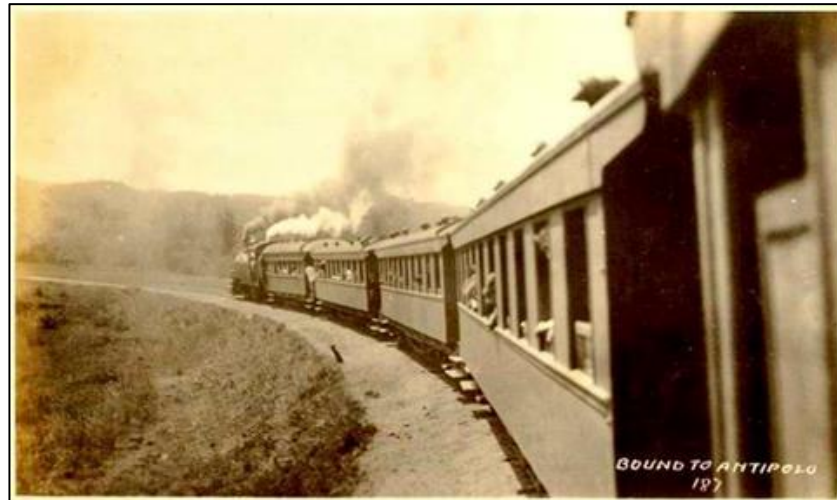
Figure 5. Manila Railroad Company train to Antipolo, Rizal
